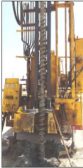
Photo (1) power drilling machine using continuous flight auger method for drilling.
